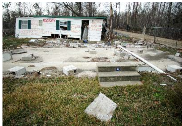
A home is knocked off its foundation by the hurricane in Mississippi. Leif Skoogfors/FEMA photo.
